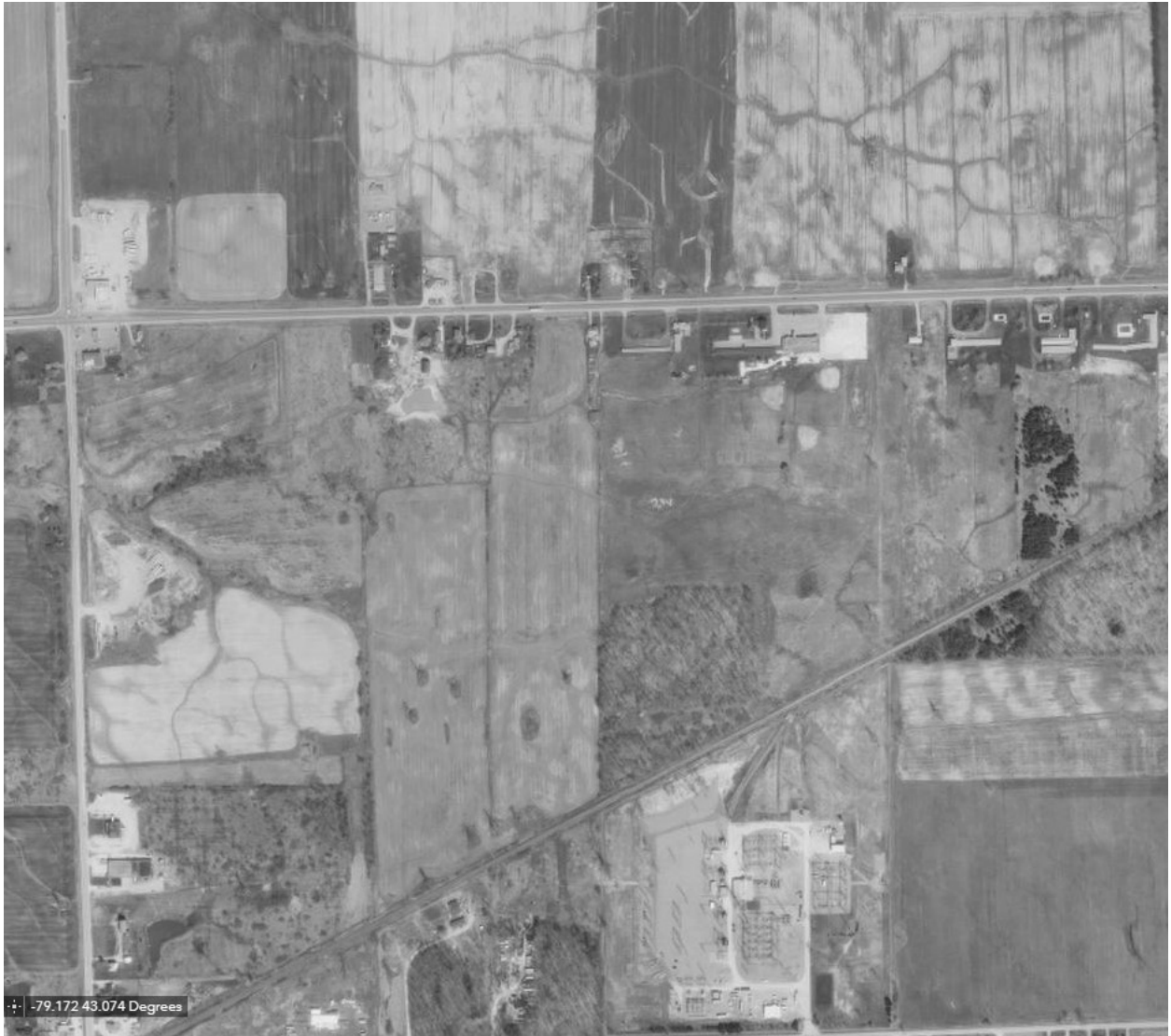
Figure 41: An overhead view of the site, circa 2000. Courtesy of the Niagara Air Photo Index.
