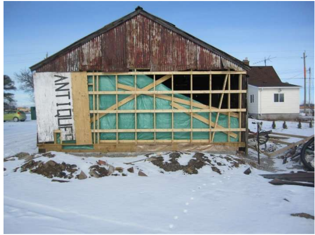
Figure 3: Rear of the building under construction
