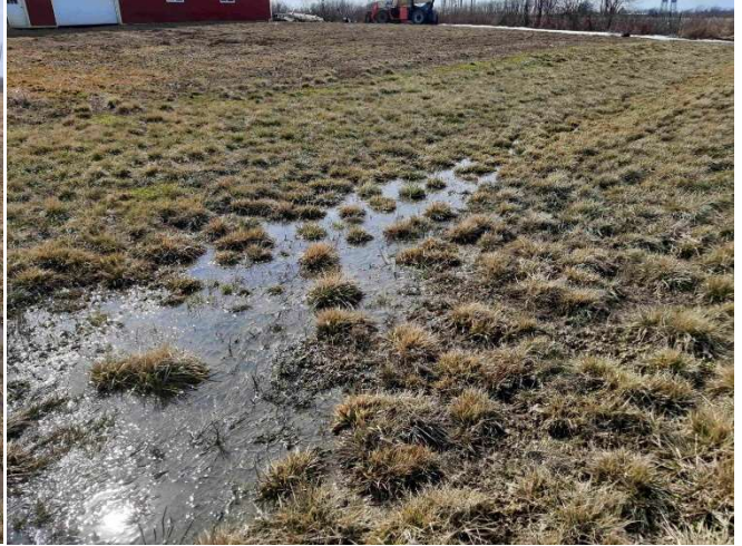
Figure 28: Western side of first flooded section
