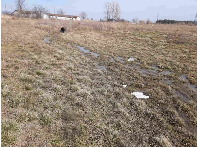
Figure 27: Eastern side of first flooded section and culvert
