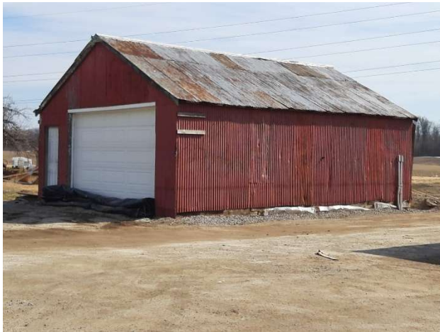
Figure 2: Building that is under construction.
