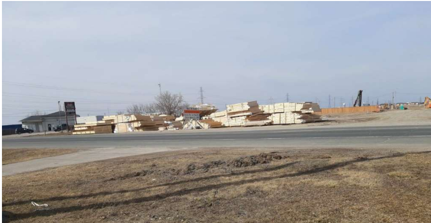
Figure 9: Lumber kept near road for sub-division construction
