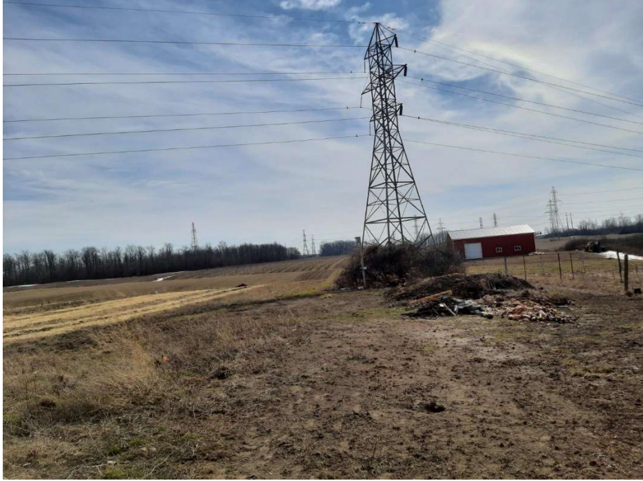
Figure 24: Transmission tower that runs the power lines through the site
