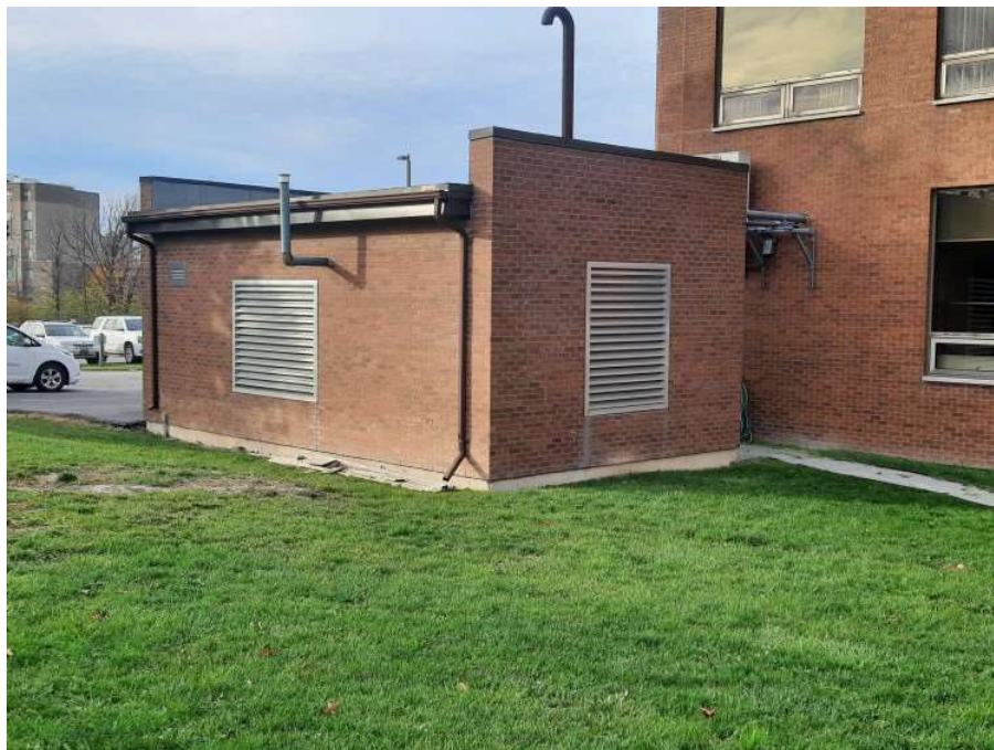
A separate small building for a diesel generator.
