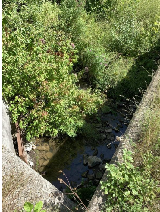
Figure 32: Site 5 (Kraft Drain)
